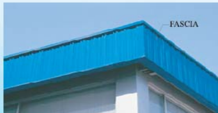
Vertical Fascia with back up panel and valley gutter
